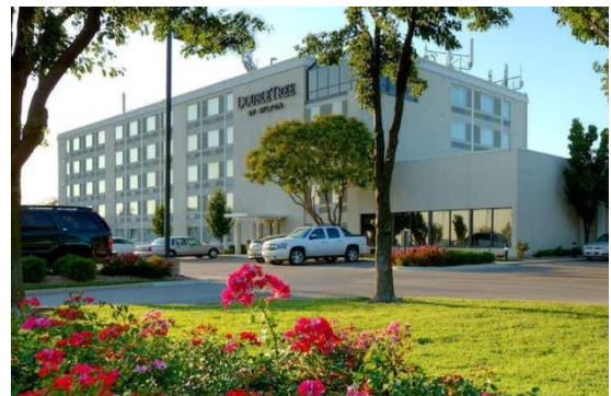
The DoubleTree by Hilton Hotel Wichita Airport
