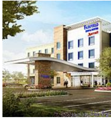
Fairfield Inn & Suites planned for Waxahachie, TX
