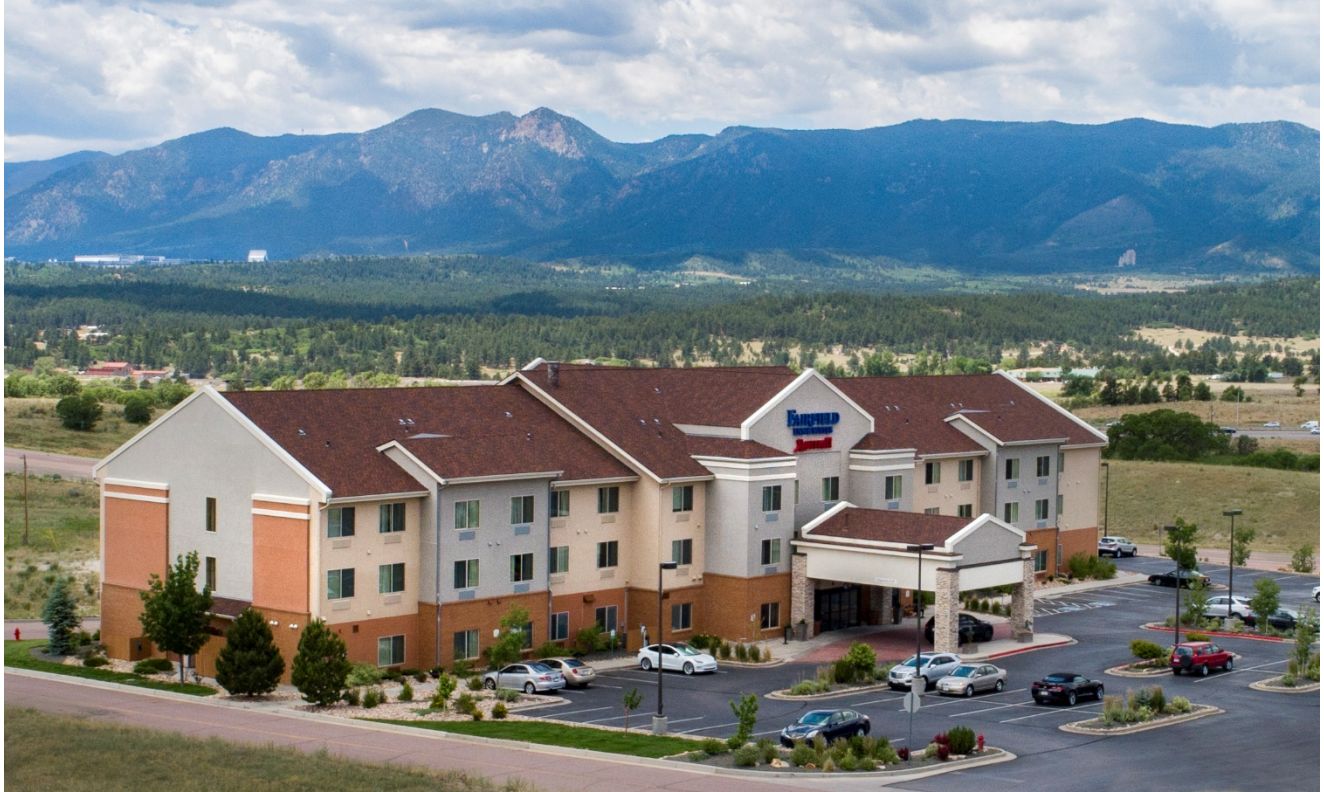
Fairfield Inn & Suites by Marriott-Colorado Springs North/Air Force Academy
